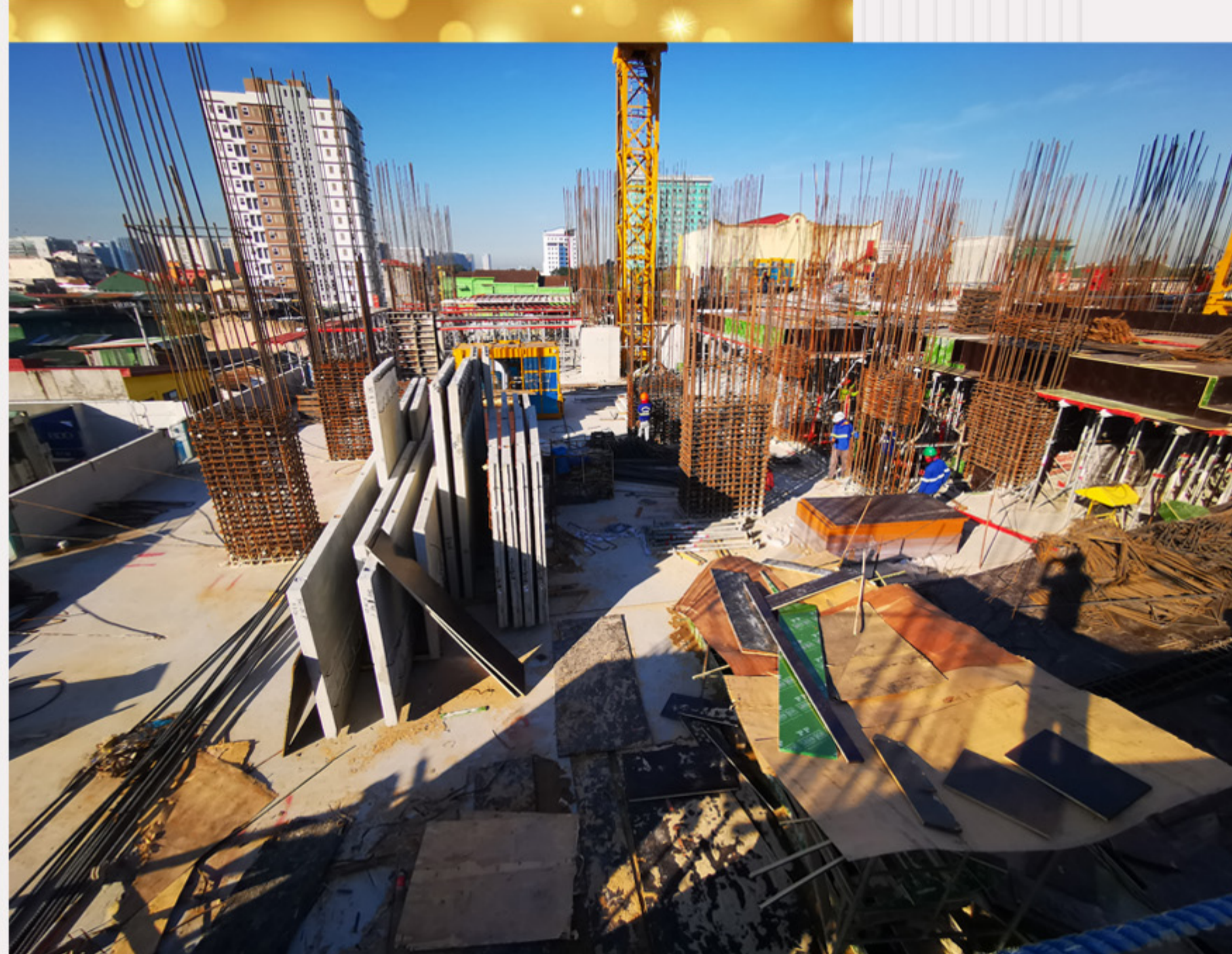
Vertical Column preparation (4th-5th floor - Zone 3) 五層立柱準備 (3區)
