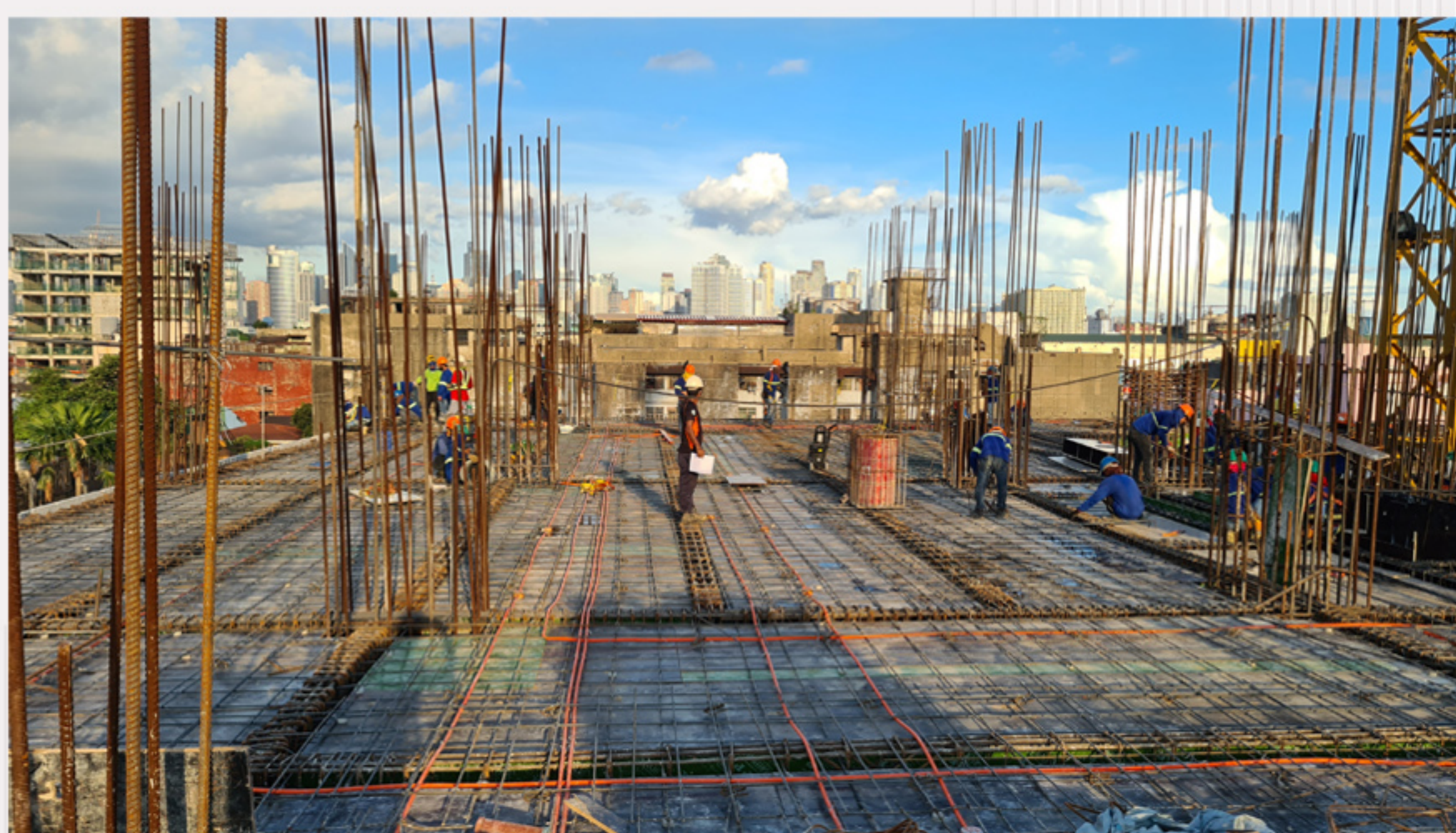
Rebar works for 5th floor slab
