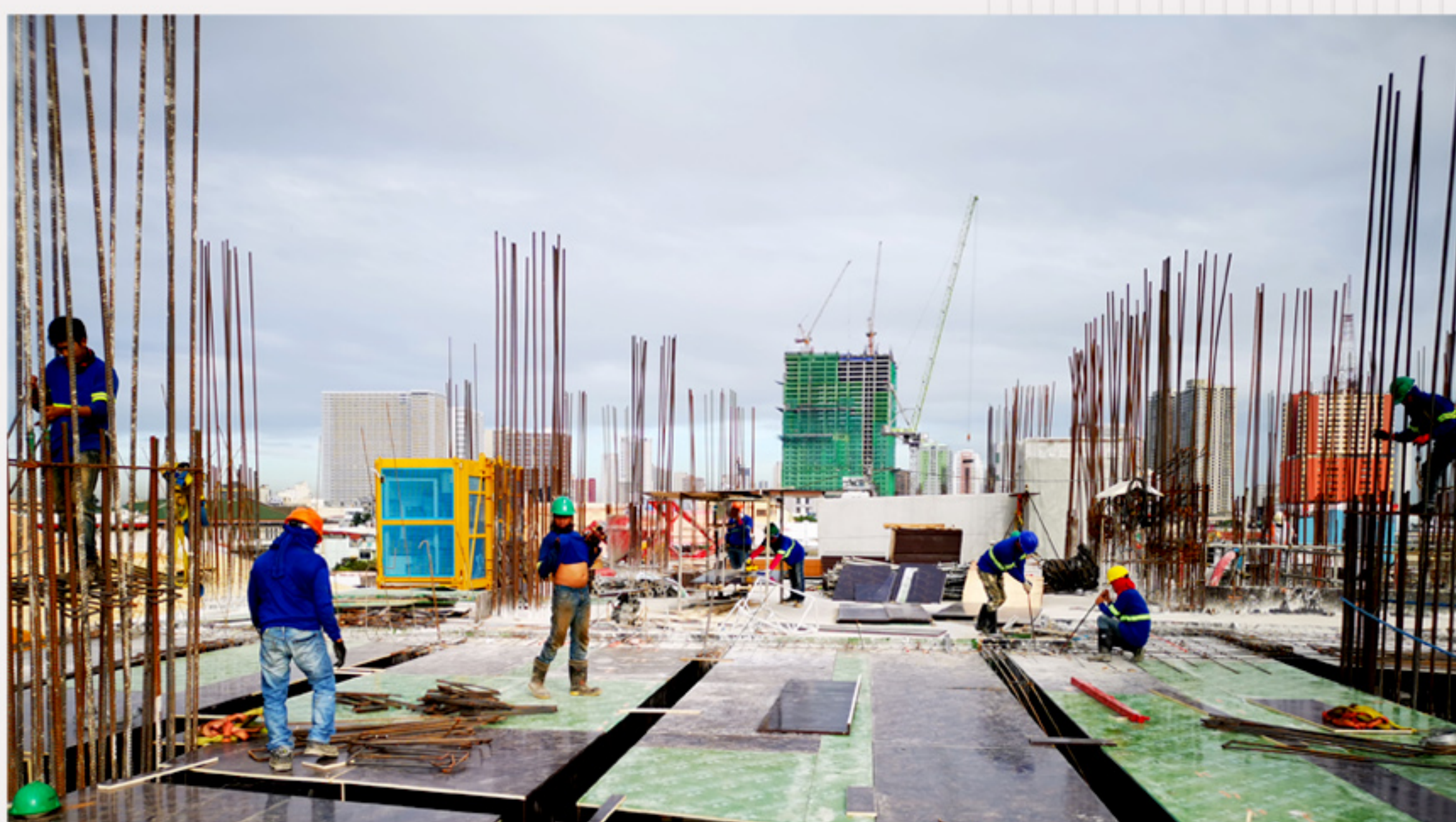
Formworks @5th floor zone 1 and zone 2
