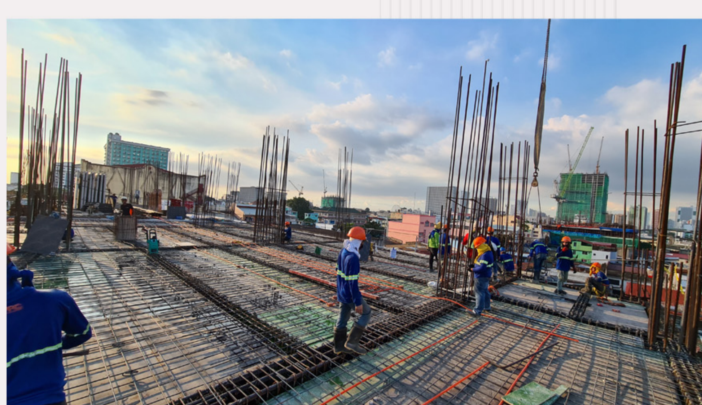
Rebar works for 5th floor slab (Zone 2) 五層樓板鋼筋鋪設 (2區)
