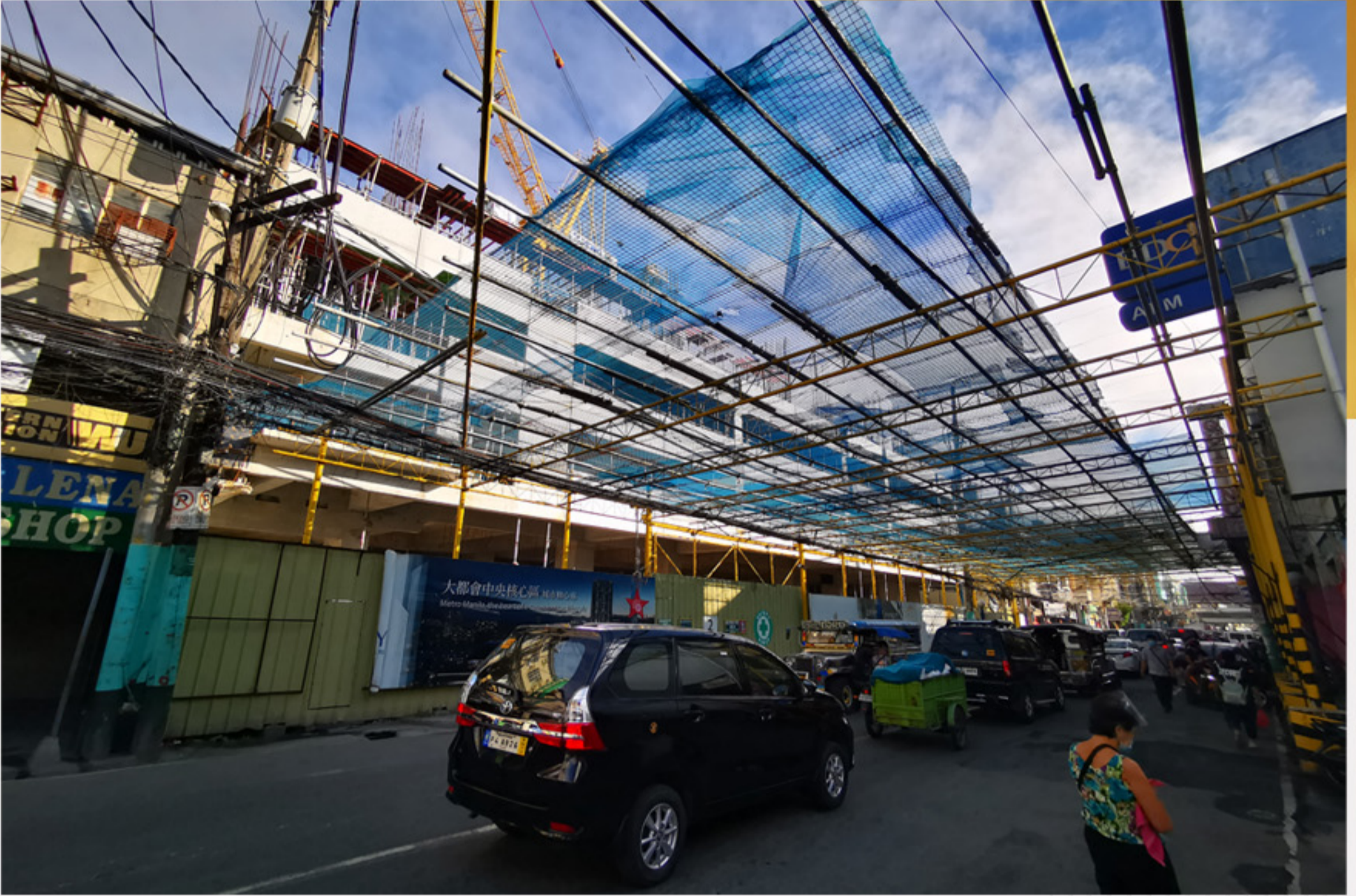
Installed street Canopy along Arnaiz Avenue 沿街外牆已安裝至四層
