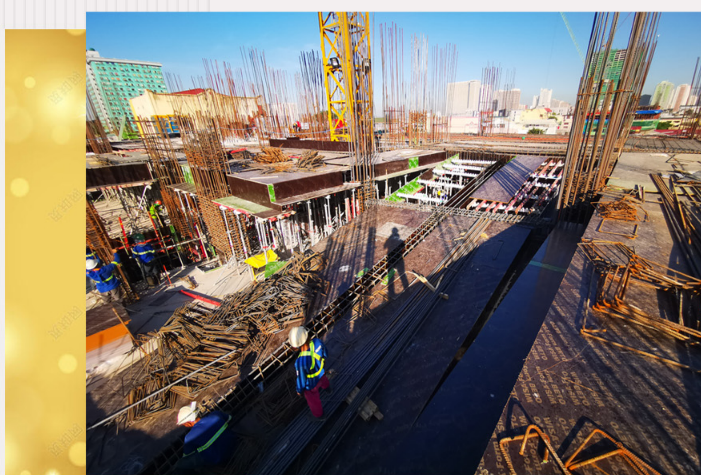
Formworks installation (Ramp 4th-5th floor) 四至五層的車道模板安裝
