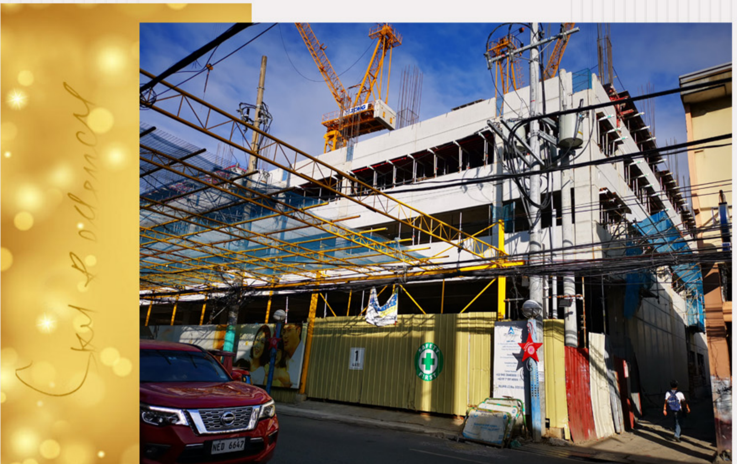
Installed street Canopy along Arnaiz Avenue 沿街外牆已安裝至四層
