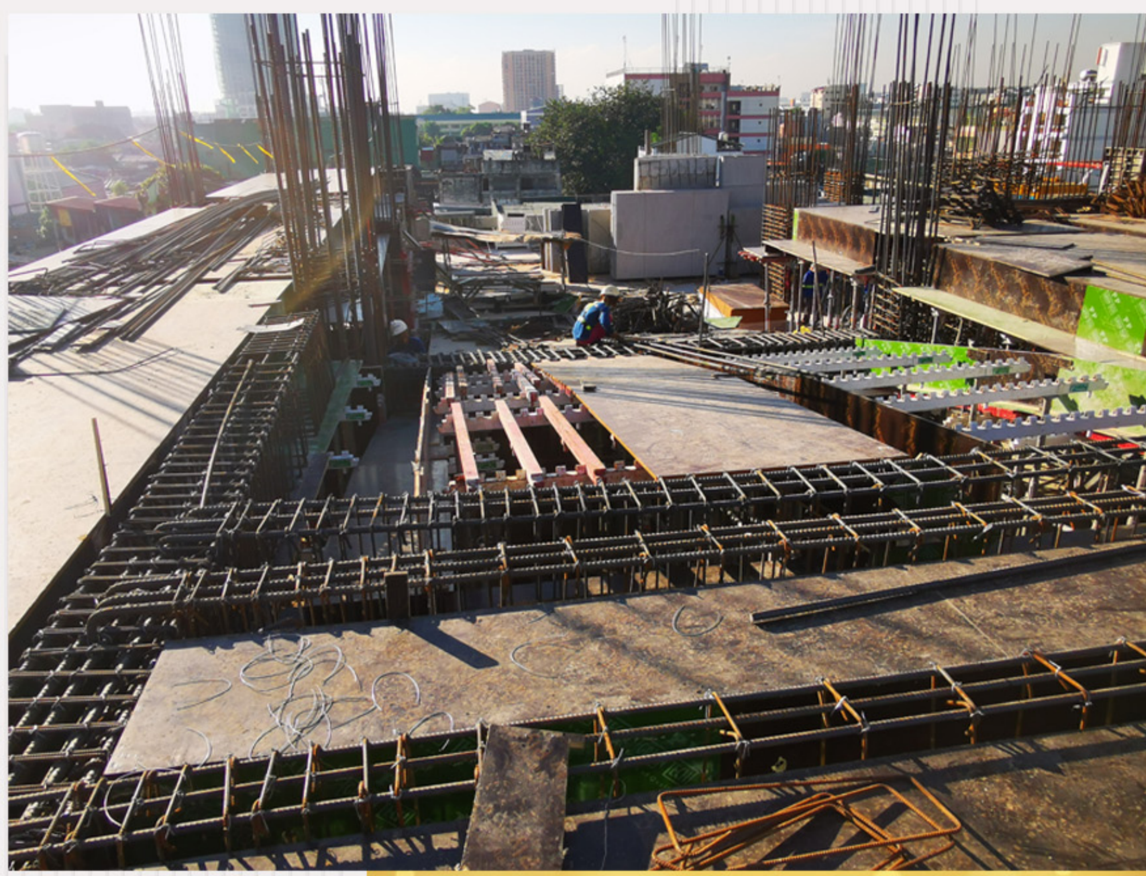
Formworks installation (Ramp 4th-5th floor) 四至五層的車道模板安裝
