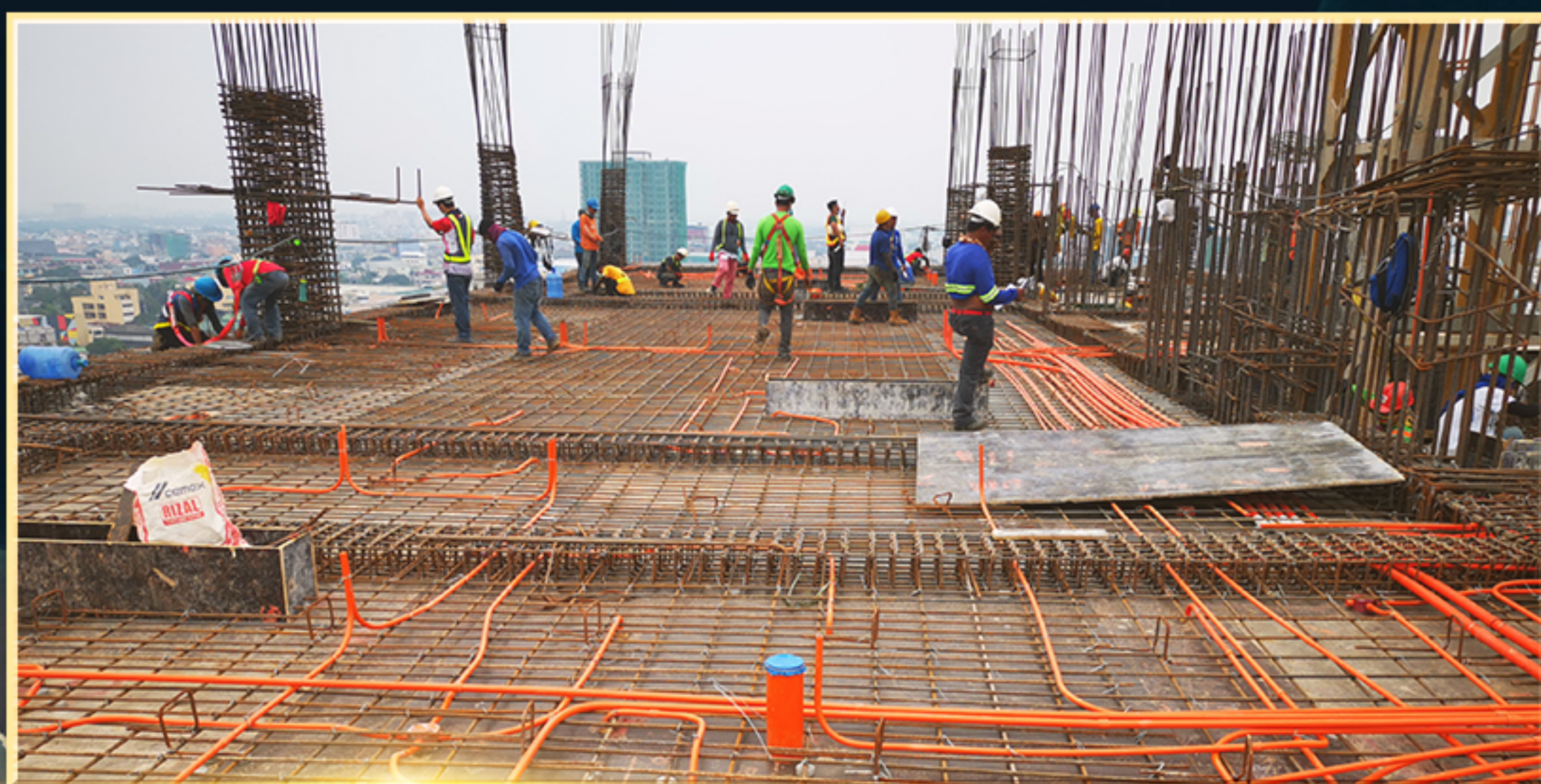
Rebar Installation (17th Floor, Zone 2 and 4)
