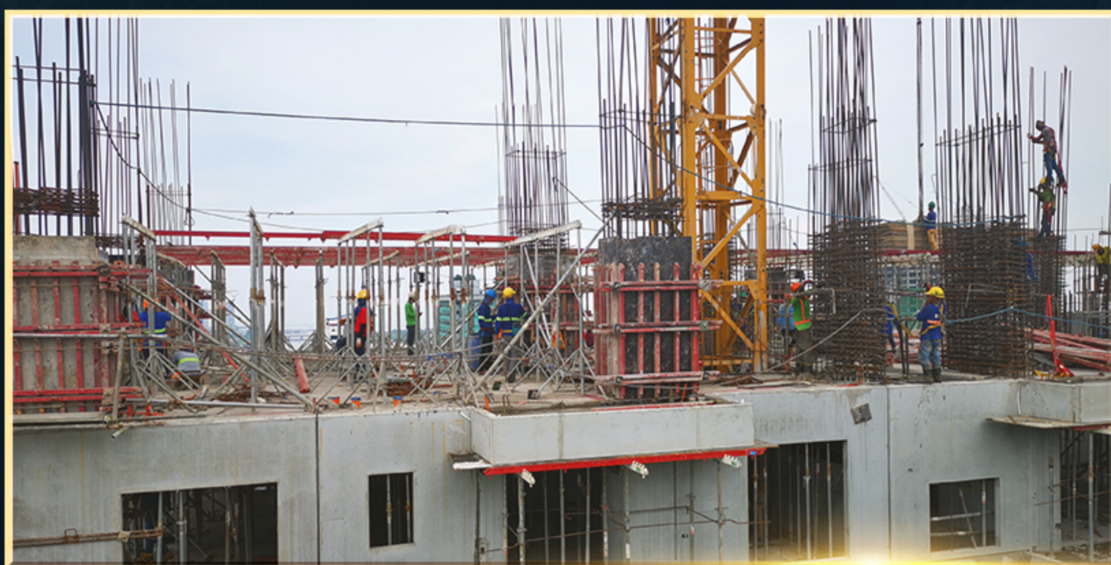
Formworks Installation (17th Floor, Zone 1 and 3)
