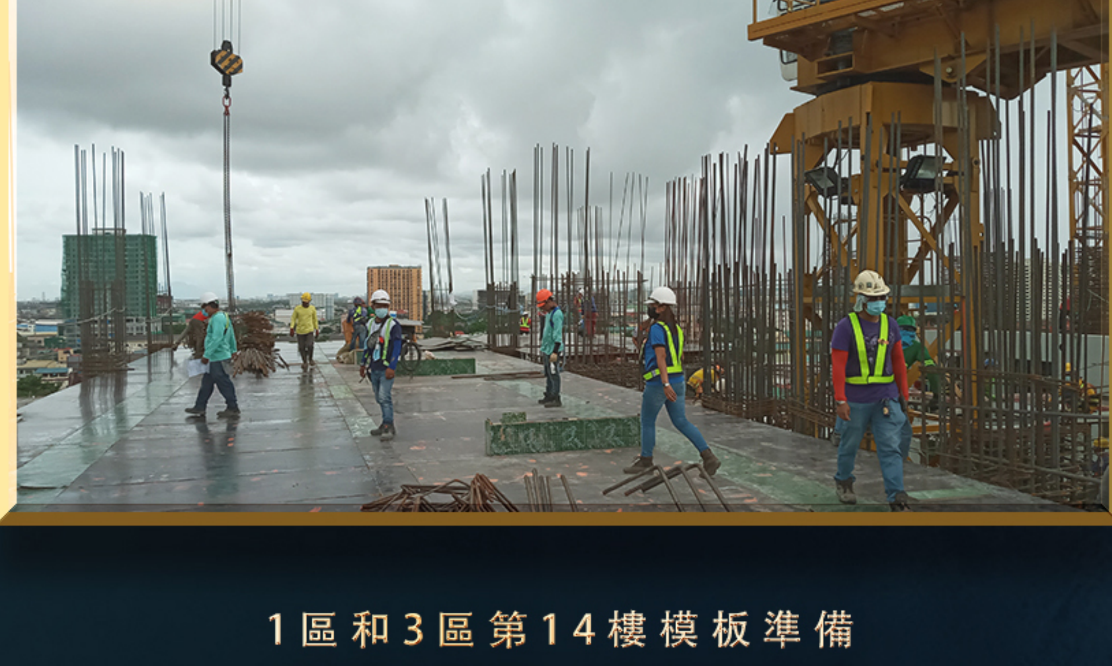
1區和3區第14樓模板準備 Formworks Preparation (14th Floor, Zone 1 & Zone 3)
