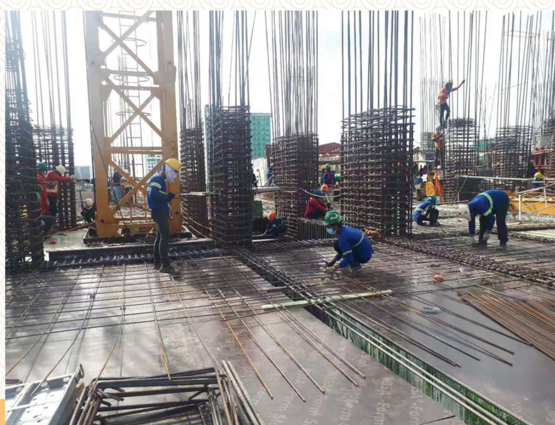
Slab Formworks and Rebar On-Going Installation Works at 6th Floor, Zone 3
