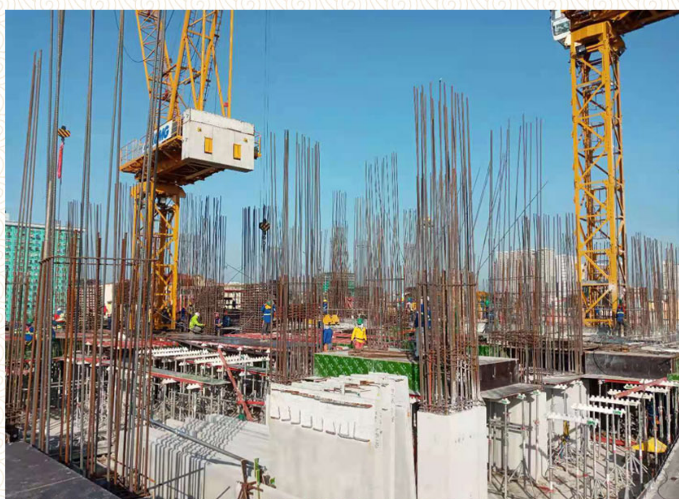
Slab Formworks and Rebar On-Going Installation Works at 6th Floor, Zone 3
