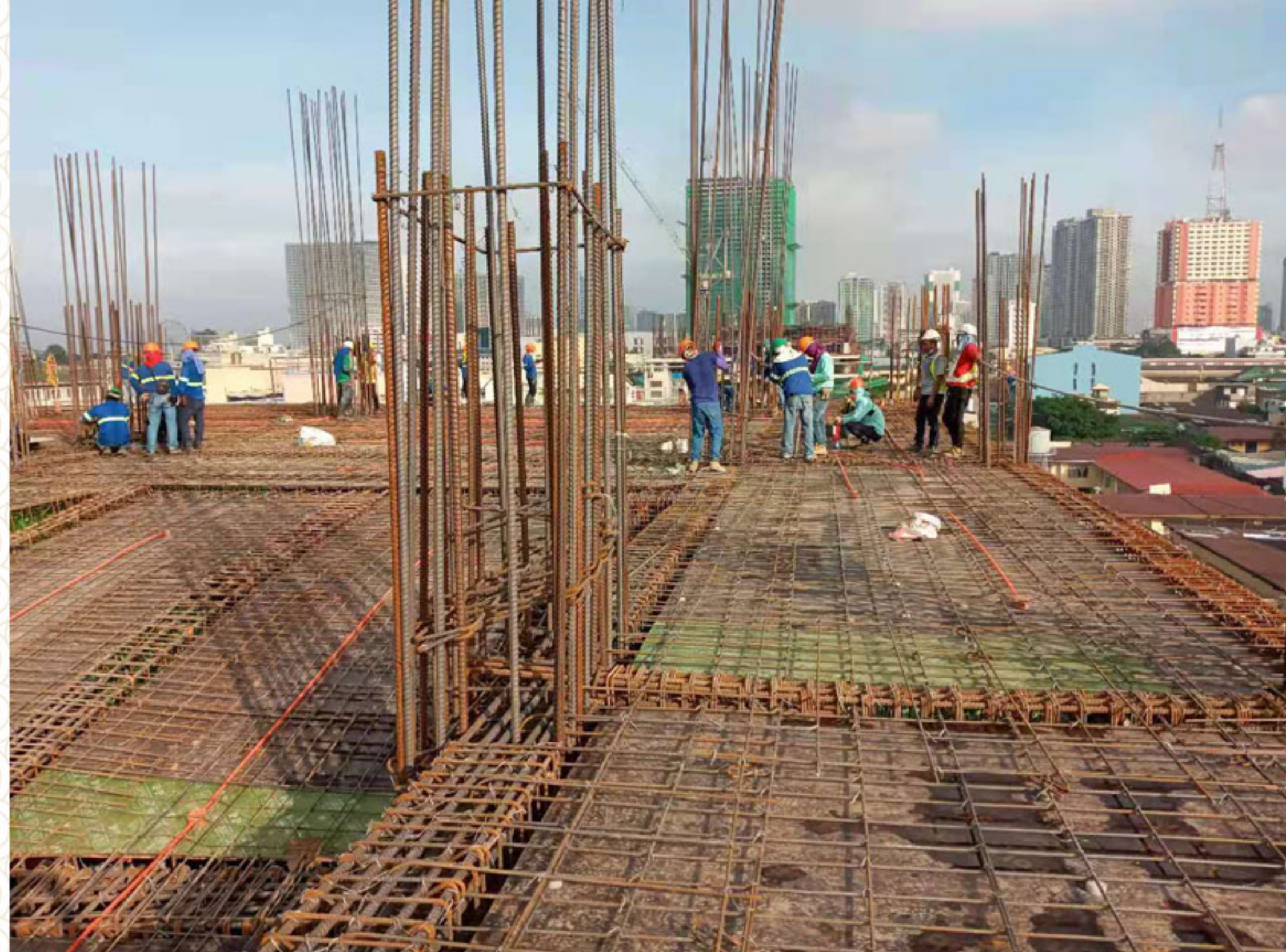
Rebar Works at 6th Floor, Zone 1.
