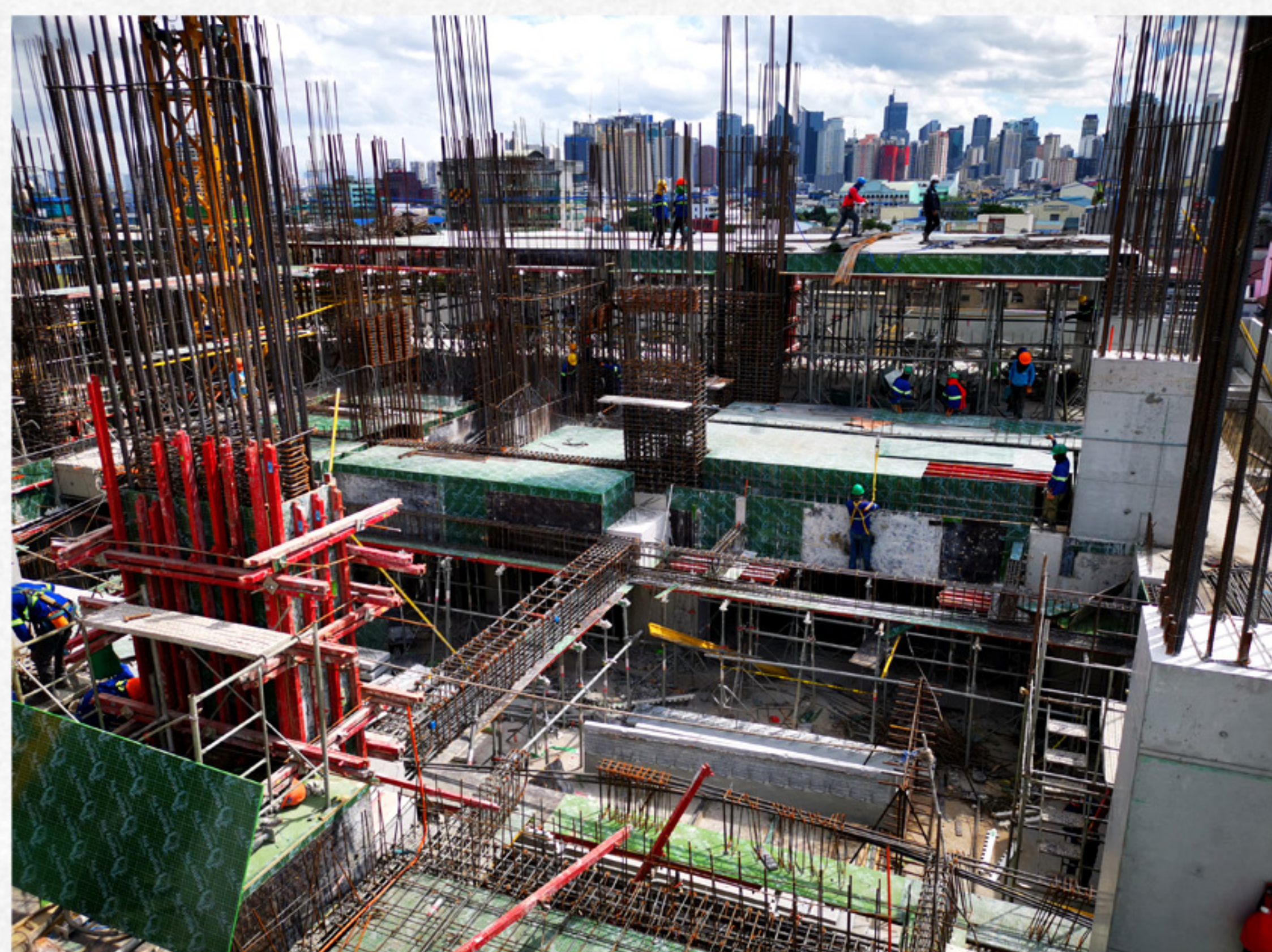
Columns and Slab Formworks at 7th – 8th Floor.
