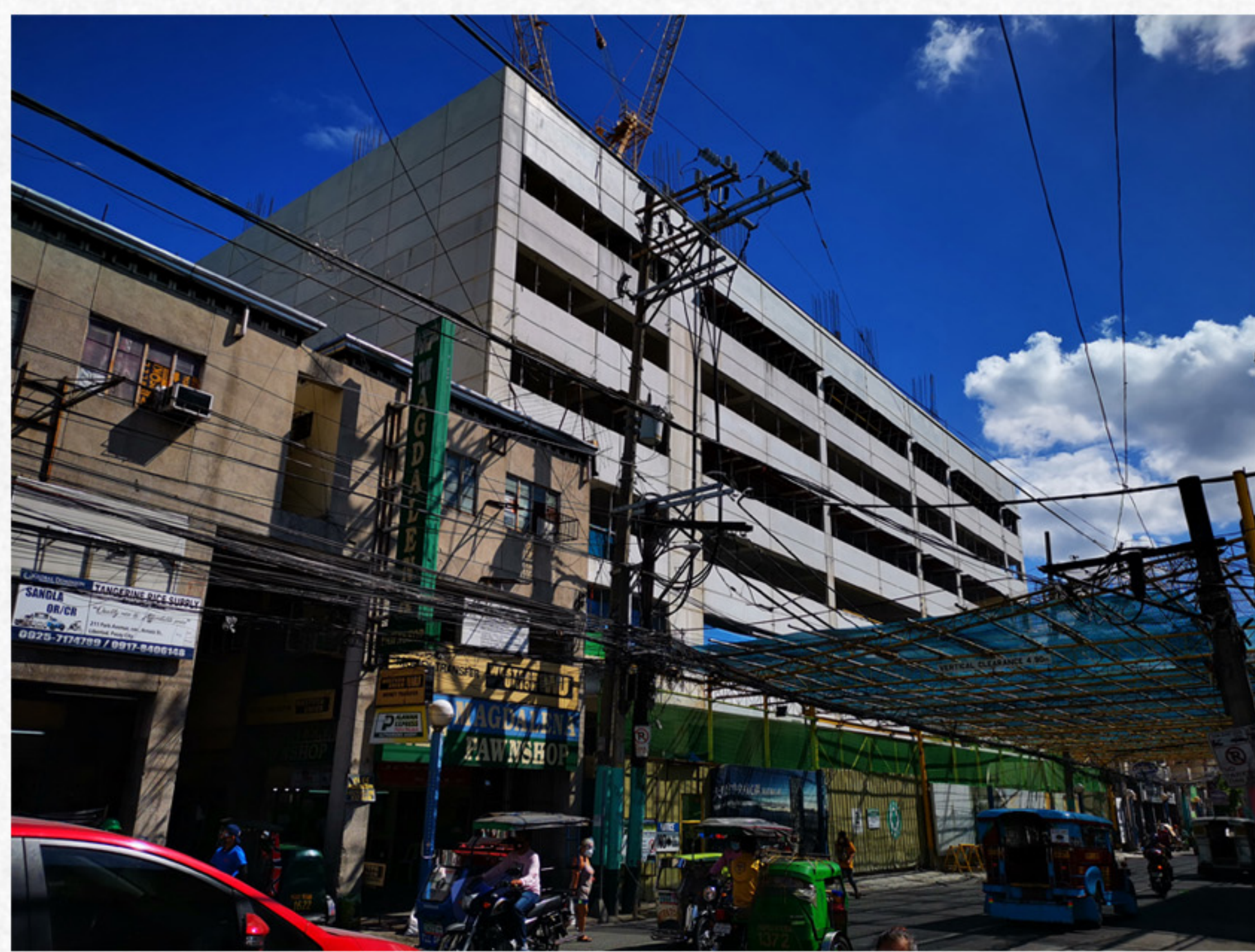
Facade Precast Wall Installation at 7th Floor Podium Parking.
